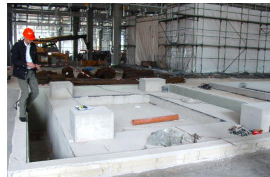
Foundation pit and foundation block
