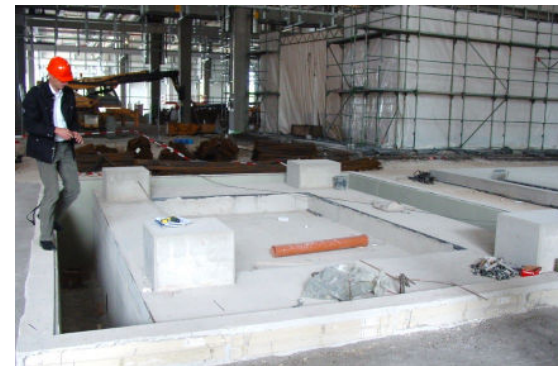
Foundation block and foundation pit
